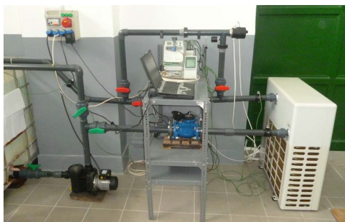
Figure 4. Heat pump measurement loop at Szent Istvan University, Faculty of Mechanical Engineering
