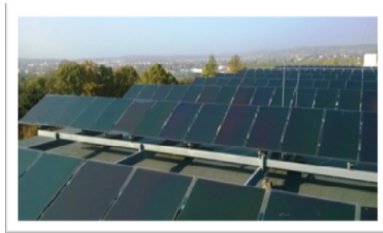
Figure 1. The picture of the studied PV system
