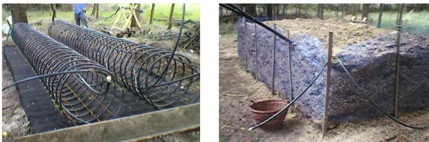
Figure 3. Installing a heat exchanger in a compost furnace
