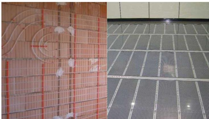
*Figure 1.* Capillary tube heat exchanger and electric heating
